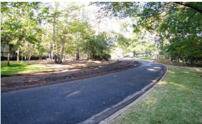
New Paving Projects
